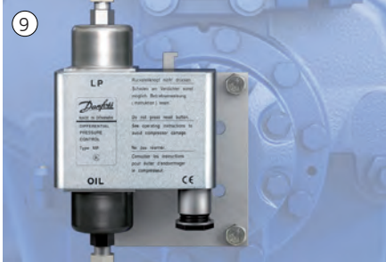
Oil pressure safety switch
